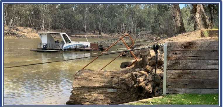
Figure 4-7 – Images showing the Structure tieback point and mooring line (Source PRS November 2024)
